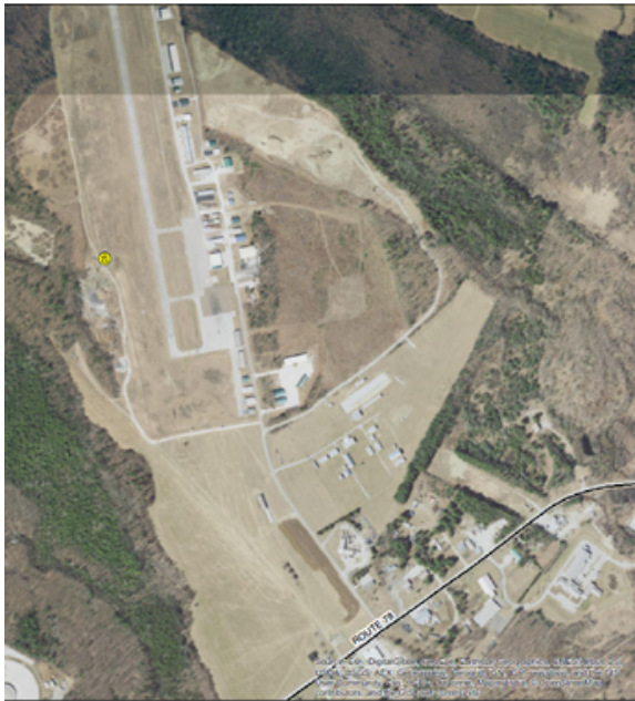
Aerial view of the airport and material stockpile location.
