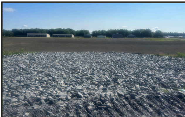
During the expansion, topsoil was stripped from the bare section above and later reclaimed with MFT.
